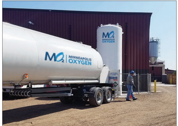
Minneapolis Oxygen filling the nitrogen bulk tank
